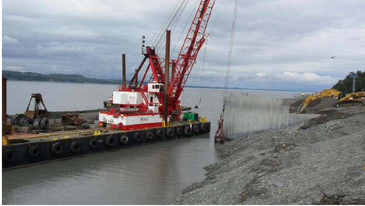
Figure 7. Manson Derrick Barge VIKING Dredging near OSCP Bulkhead
