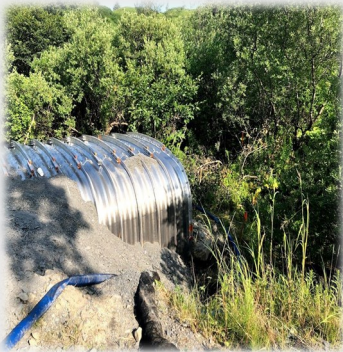
Fish passage restoration on the Buskin River in Kodiak, AK.
