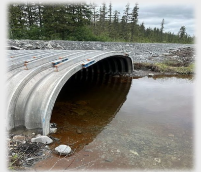
Completed fish passage culvert replacement on the Cordova Highway in Cordova, AK.
