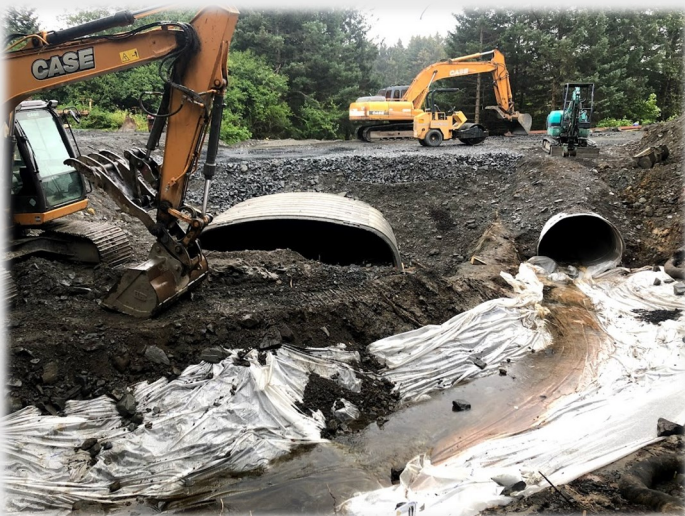
Fish passage restoration project under construction on the Buskin River in Kodiak, AK.
