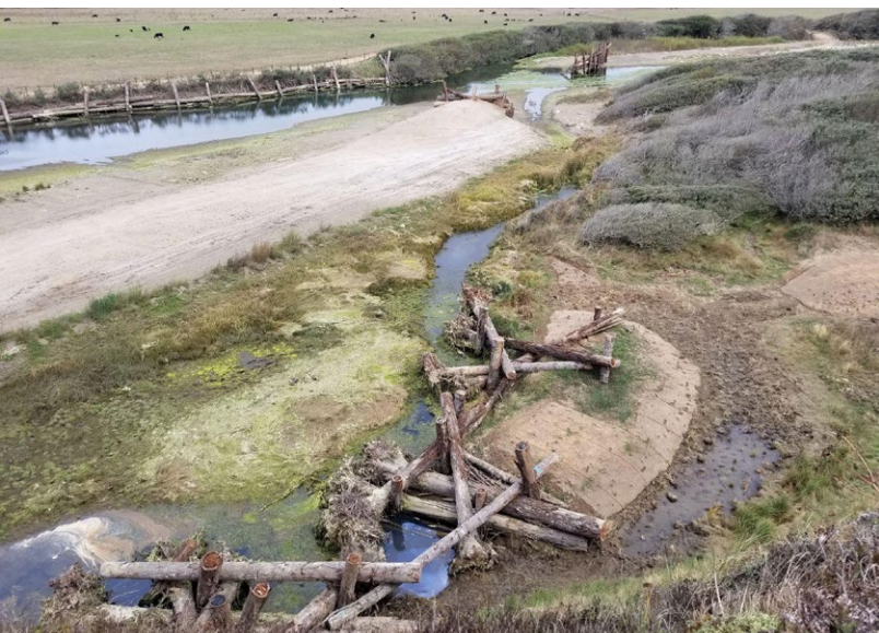
Restoring the Garcia River Estuary with large wood structures and off-channel wetland ponds (left) and a close-up (right). Credit: The Nature Conservancy
