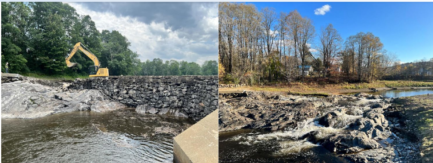
In 2022, the Atlantic Salmon Federation removed the Walton's Mills Dam on Temple Stream in the Sandy River watershed, which improved access to 40 miles of juvenile salmon rearing habitat. Credit: Atlantic Salmon Federation
