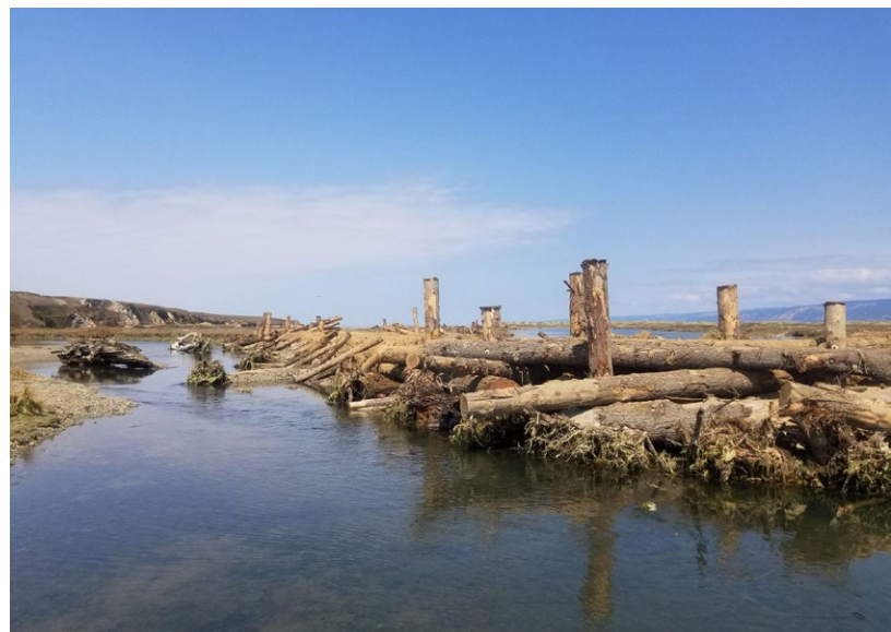
Restoring the Garcia River Estuary with large wood structures and off-channel wetland ponds (left) and a close-up (right). Credit: The Nature Conservancy
