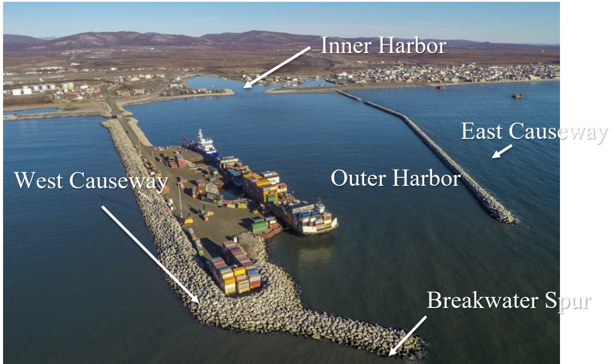
Figure 1. Aerial Overview of Port of Nome on Norton Sound, Bering Sea, Alaska.
