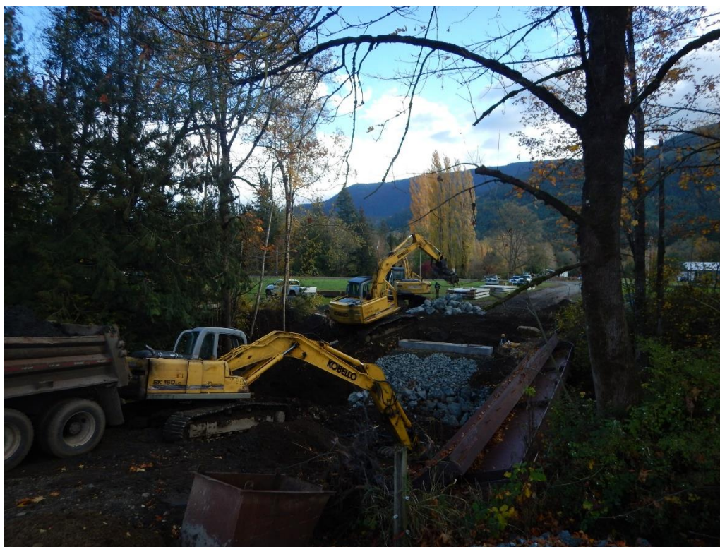
Photo: Culvert replacement for fish passage restoration. Credit: Nooksack Salmon Enhancement Association.
