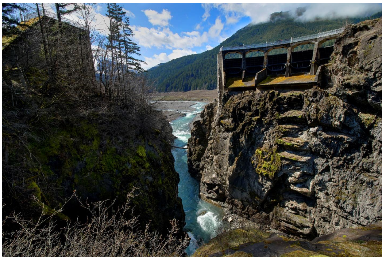
Photo: Elwha River flowing through the former site of the Glines Canyon Dam. Credit: ©John Gussman (used by agreement).
