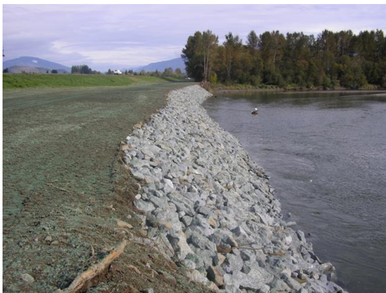
Photo: Skagit River levee isolating the river from the floodplain. Credit: NMFS.
